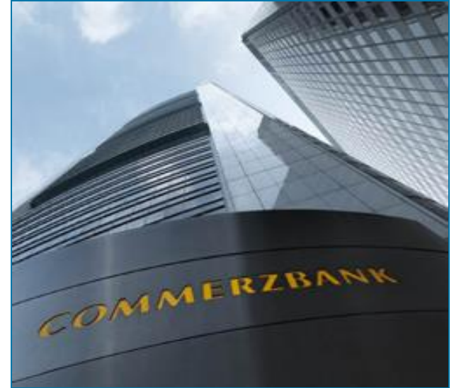
Commerzbank headquarters in Frankfurt.
