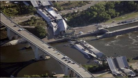
I-35W Bridge, US (2007)
