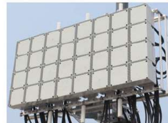
Massive MIMO antenna array for a Huawei 5G field trial.
